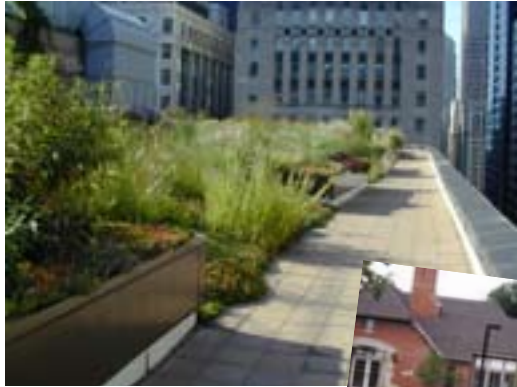
(Above) Green roofs are recommended to help reduce water runoff. (Right) Underground storm water management systems are appropriate for urban areas.
