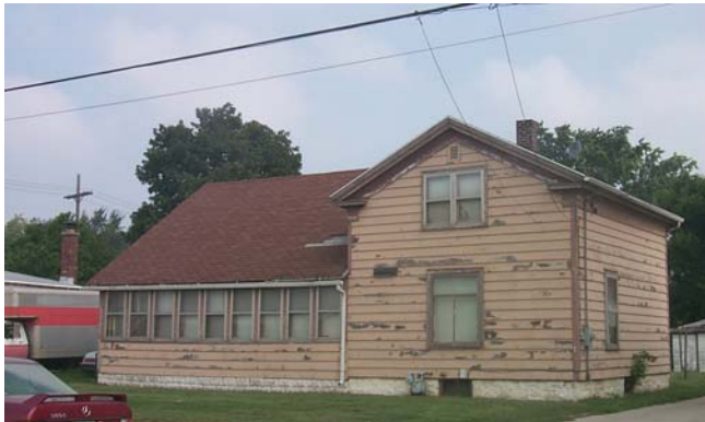
Before – Owner completed roof replacement using private investments.
