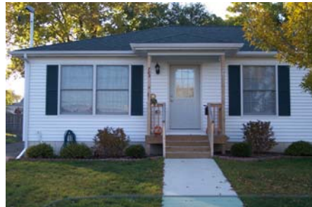
After – Three-bedroom home, constructed with private funds, improved the appearance of the neighborhood and increased the affordable housing stock.
