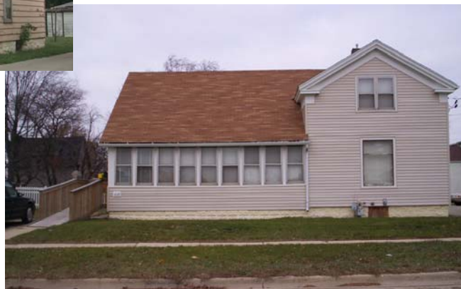
After – City funded the installation of the siding and accessible ramp.
