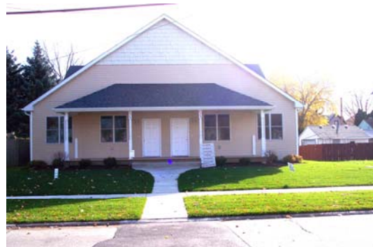
After - Front of new two-family home. Constructed with private investment.
