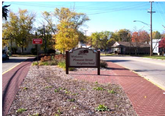
After – Completed entryway to the neighborhood.
