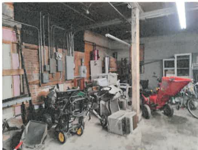
REAR GROUND FLOOR STORAGE
