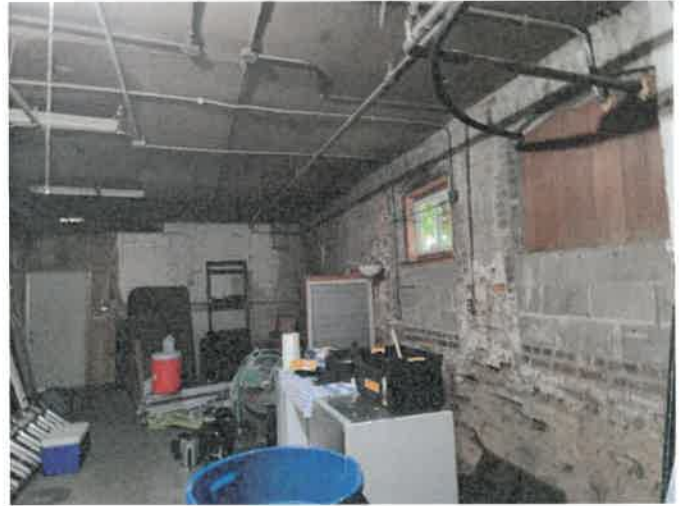
REAR GROUND FLOOR STORAGE
