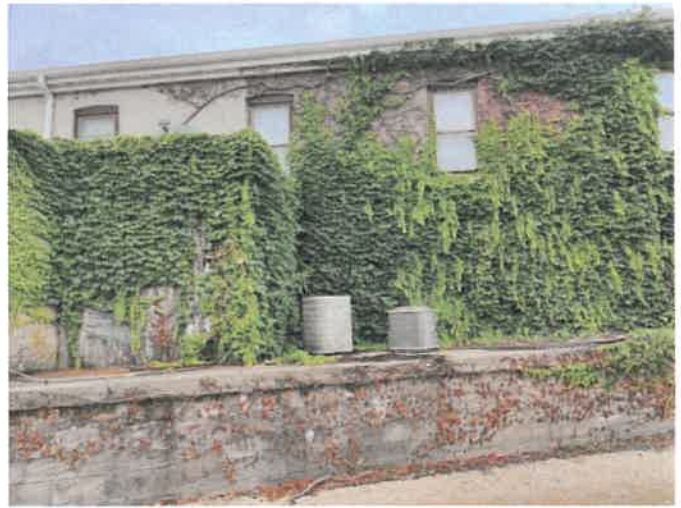
TWO-STORY SECTION - SOUTH FAÇADE
