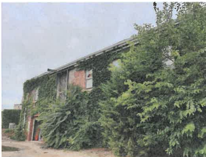
TWO-STORY SECTION - SOUTH FAÇADE
