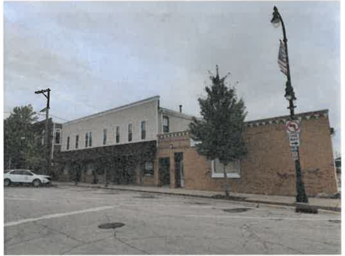
FRONT (WEST) FAÇADE
