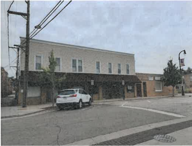
FRONT (WEST) FAÇADE
