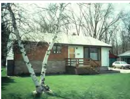
Home elevated one foot above the base flood elevation.
