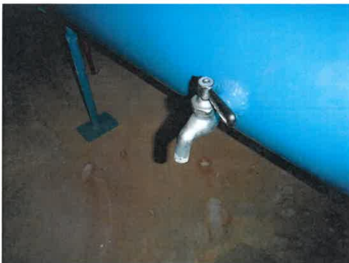
69) There is a sample tap on the fill/draw pipe in the building.
