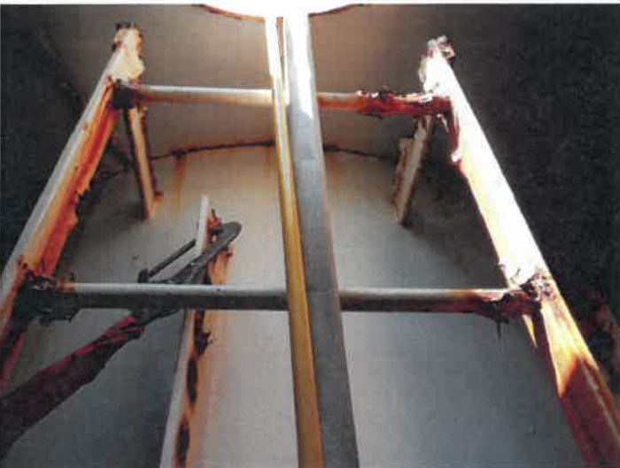
54) There is steel loss from corrosion on the wet interior ladder above the high-water level.
