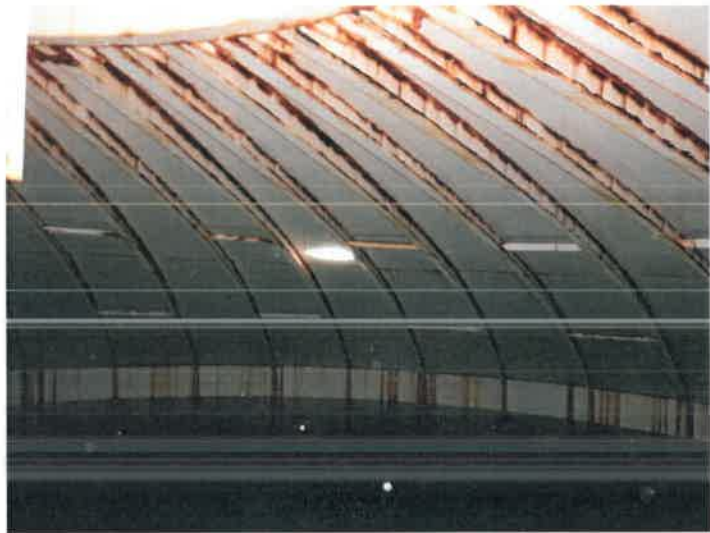
50) Coating failures on the wet interior roof.
