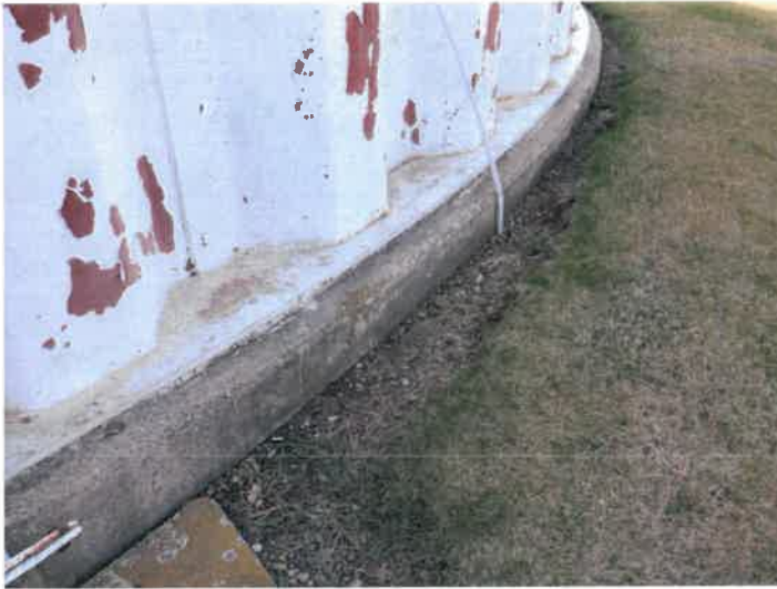
1) Minor crack in the concrete foundation.
