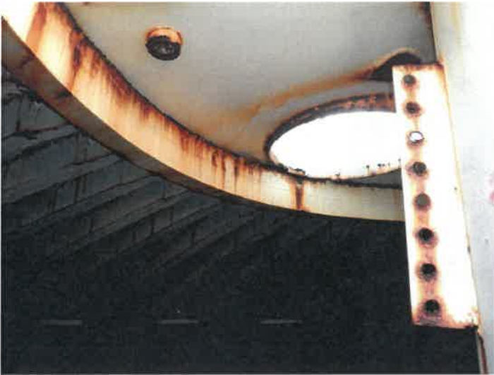
52) Spot coating failures and minor corrosion on the wet interior roof.
