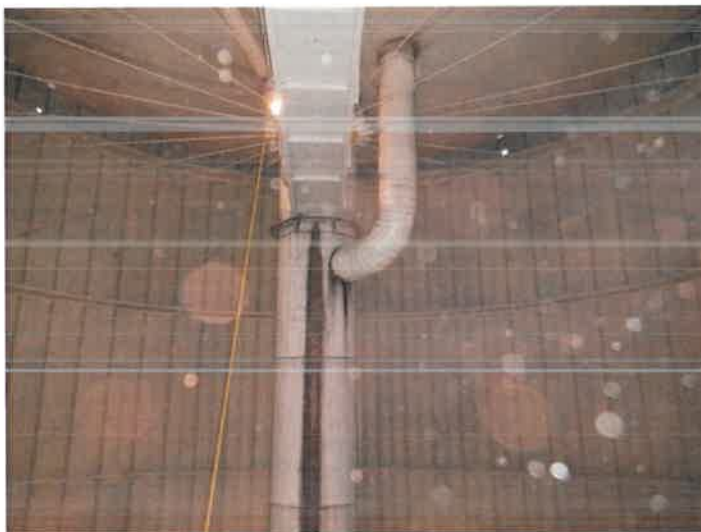
39) The 5 foot wet riser ends below the top platform and there is a separate pipe from it that fills/draws from the tank.
