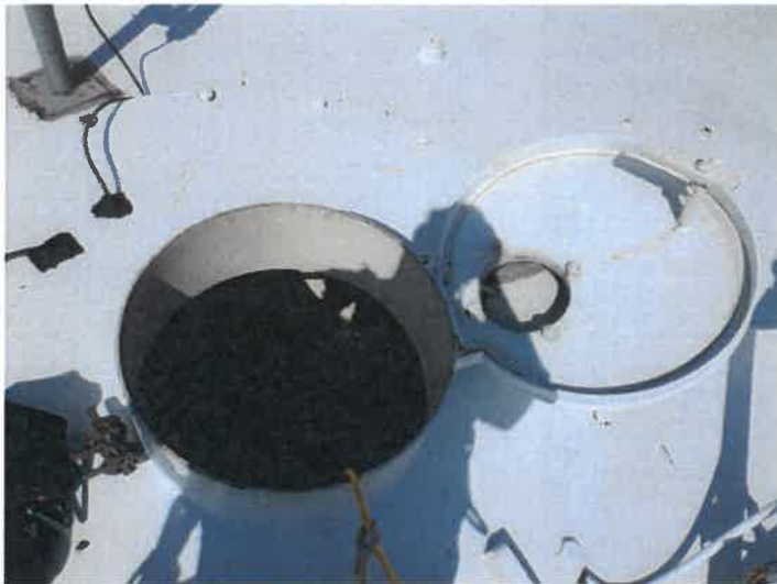
28) The access tube hatch is in fair condition.
