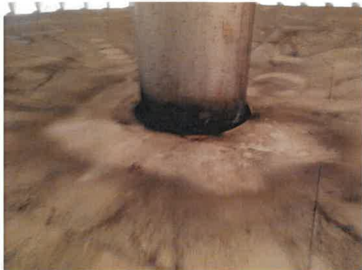
35) Spot coating failures on the condensate platform.
