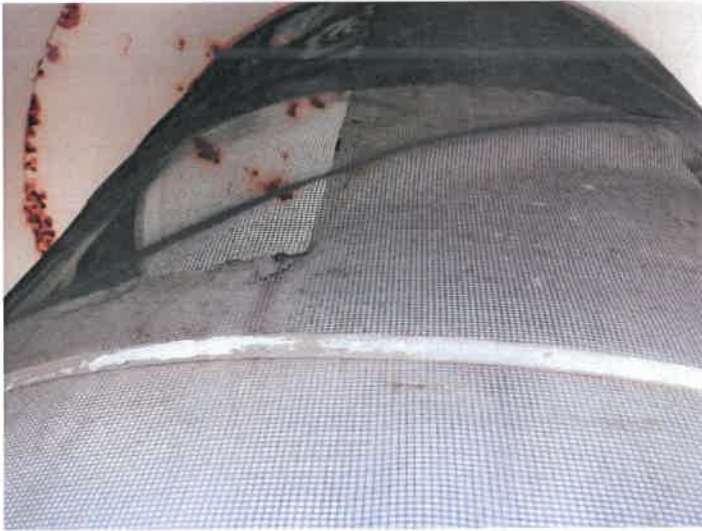
25) The roof vent screen is in good condition but is oversized.
