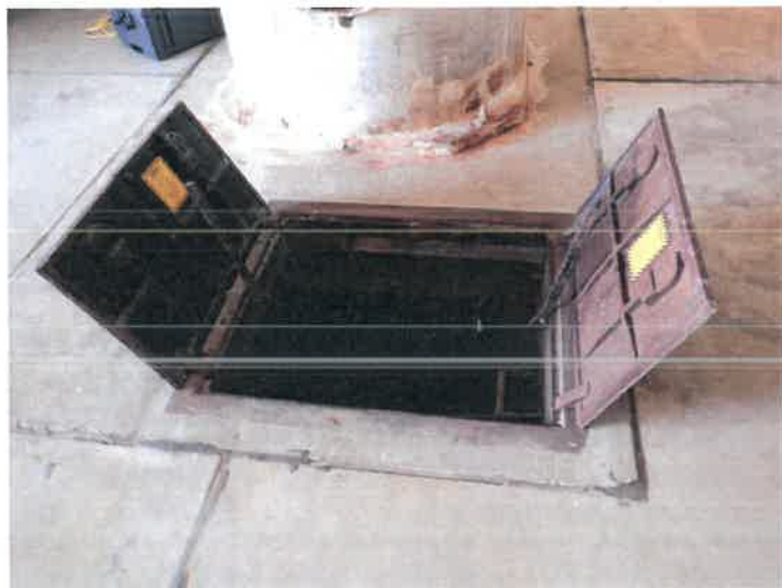
68) There is a metal cover to the pit that is in fair condition.
