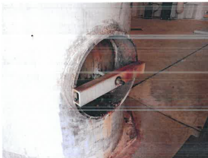
33) The manway in the wet riser is in good condition. The coating is in fair condition.
