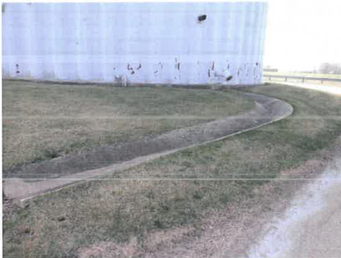
9) The overflow discharge area is in good condition.
