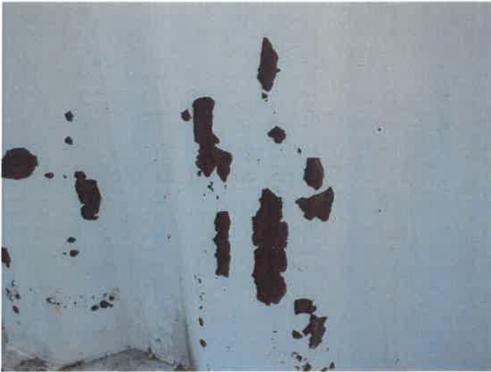
4) Coating delamination on the column.
