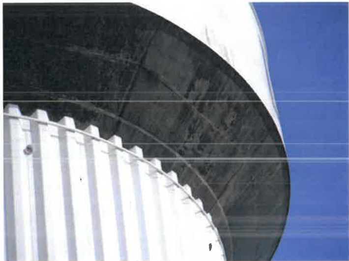
14) There are spot coating failures on the bowl. The bowl is covered with mildew.
