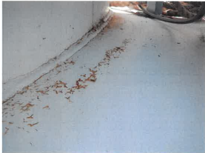
23) Rust undercutting on the roof coating near the vent.
