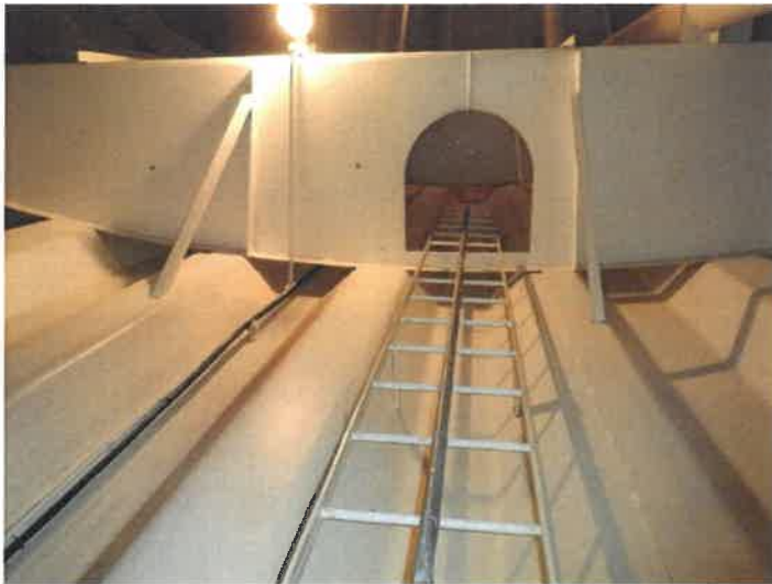
40) The dry interior column ladders above the condensate platform are in good condition.
