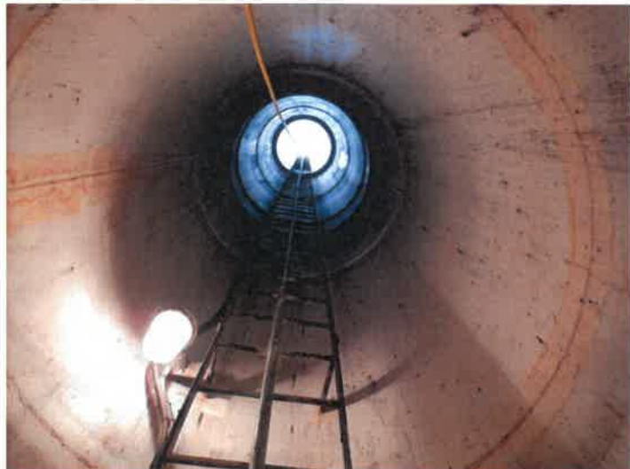
47) The access tube coating is in poor condition overall.
