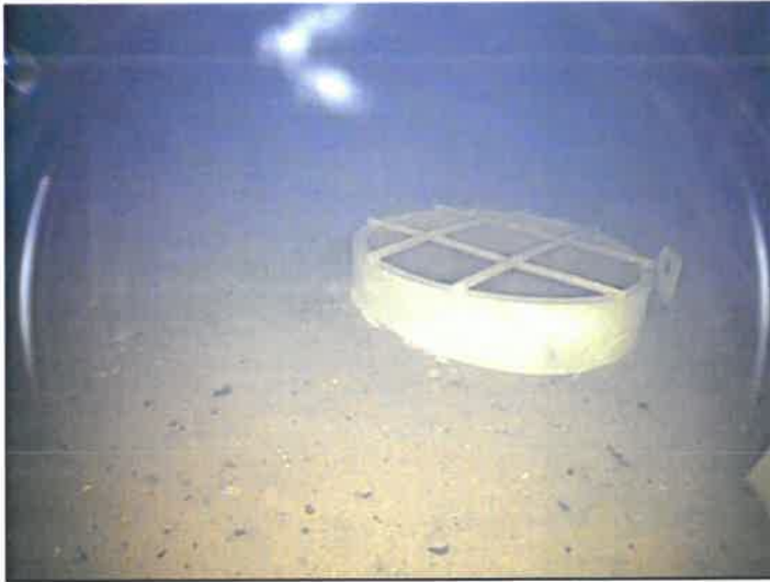
67) The fill/draw pipe is in good condition.
