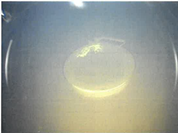
66) The wet interior manway cover is in good condition.
