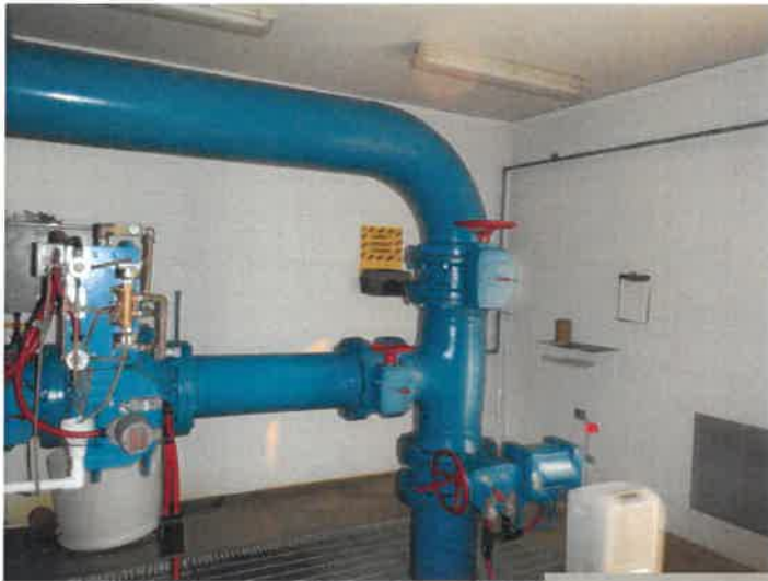
67) Coating on the piping in the building is in good condition.
