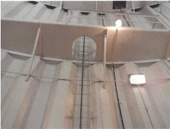
34) The dry interior column ladders below the top platform are in good condition.
