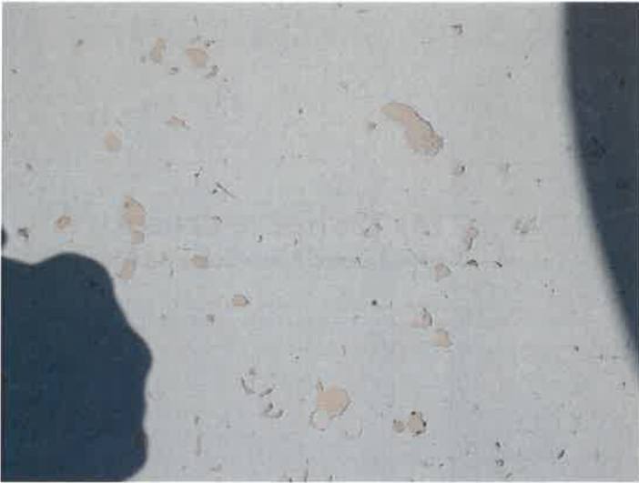
22) Topcoat delamination on the roof.
