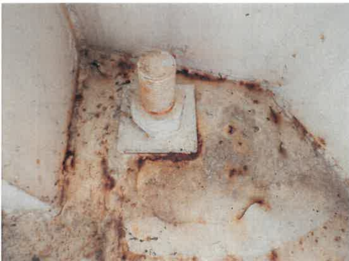
30) The anchor bolts in the dry interior are in good condition.
