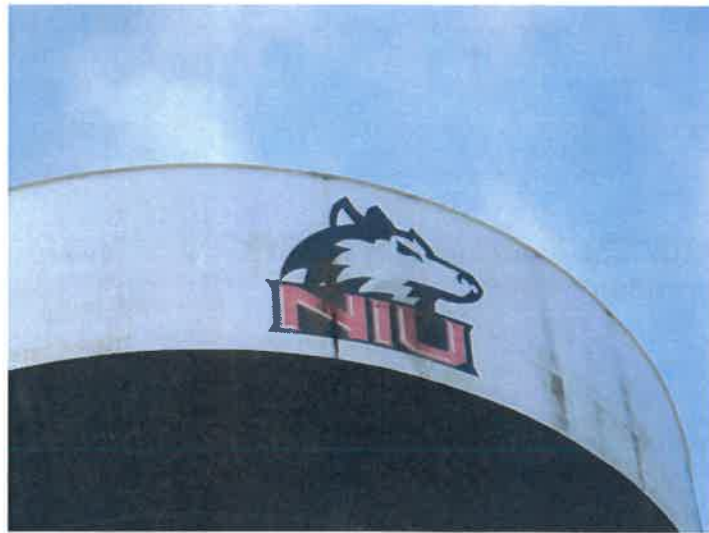
17) The sidewall coating has faded
