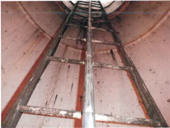
49) Spot coating failures on the access tube ladder.
