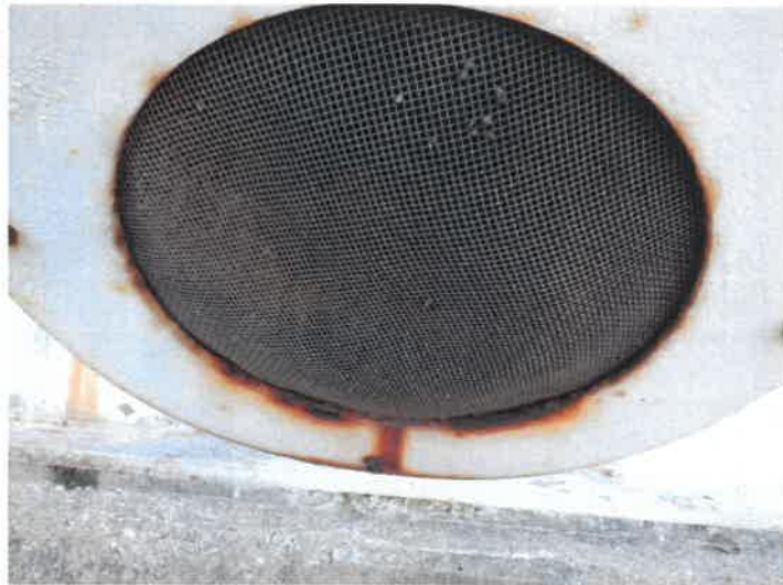
11) The screen on the overflow discharge is in good condition but is oversized.
