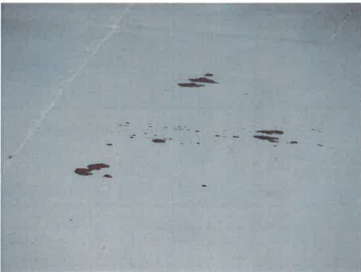
18) Coating delamination and spot coating failures on the roof.
