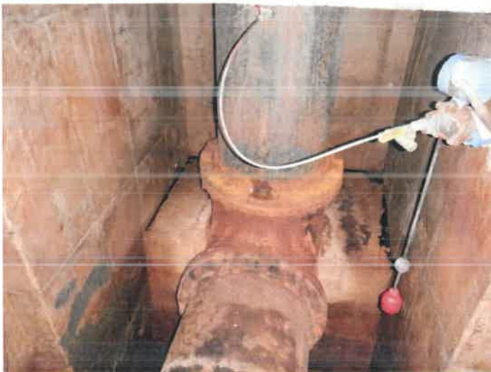
69) Coating on the pit piping is in poor condition.
