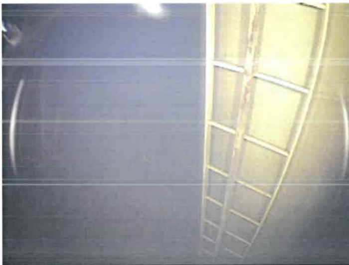
63) The wet interior ladder is in fair condition.
