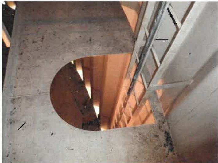
41) There is no cover over the hatch in the top platform.
