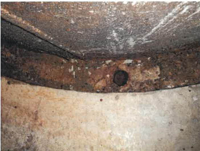
36) Coating failures around the condensate drain.
