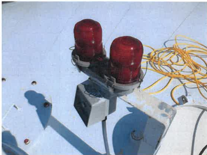
29) The double aviation light appears to be in good condition but did not operate during the inspection.
