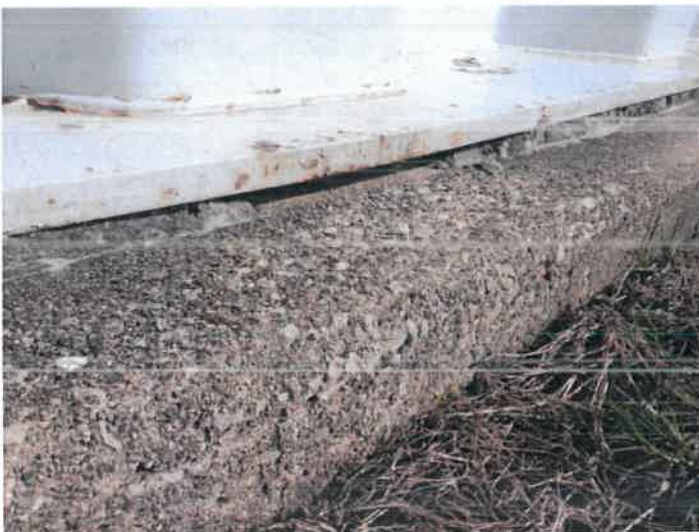
3) Missing grout between the tank baseplate and foundation.
