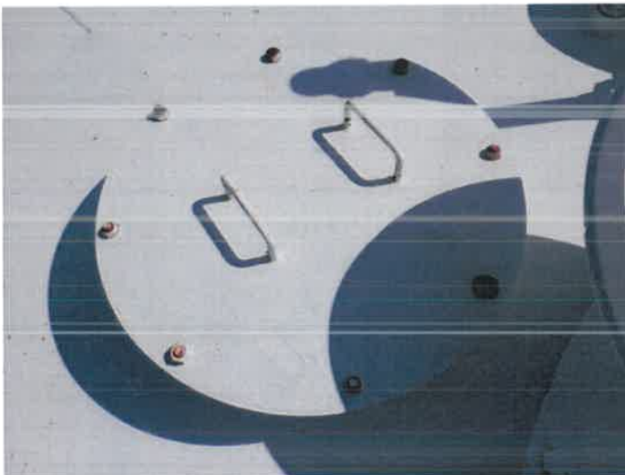
27) The bolted ventilation hatch is in good condition.
