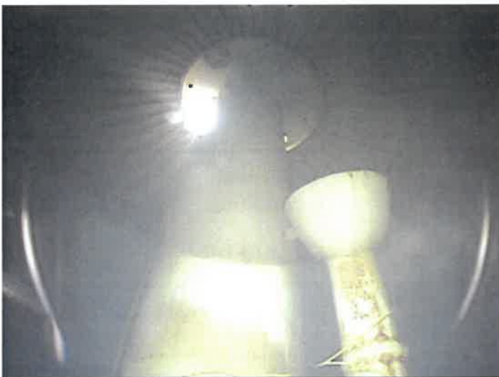
60) Spot coating failures on the upper access tube and overflow pipe.
