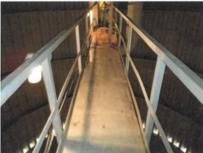
42) Spot coating failures on the top platform.
