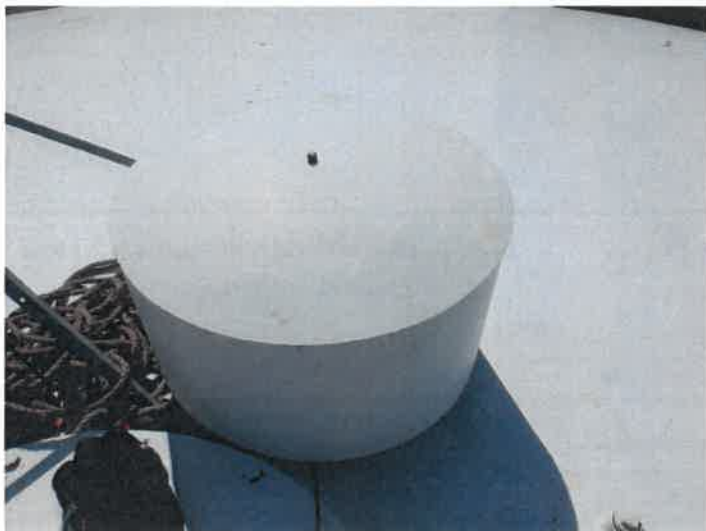
24) The roof vent is in fair condition.
