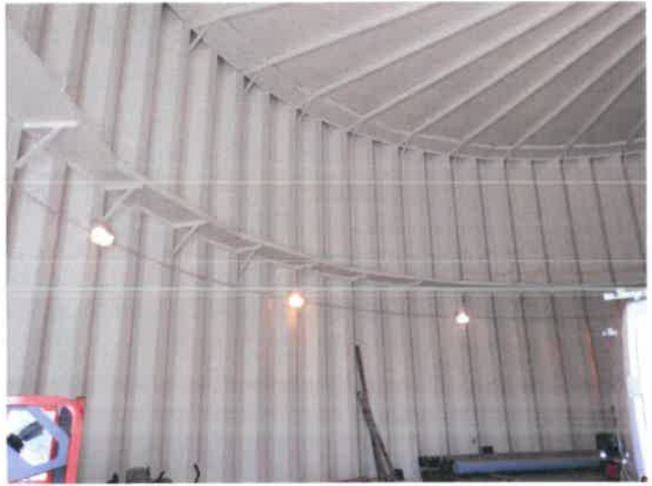
32) The dry interior column coating below the condensate platform is in good condition.
