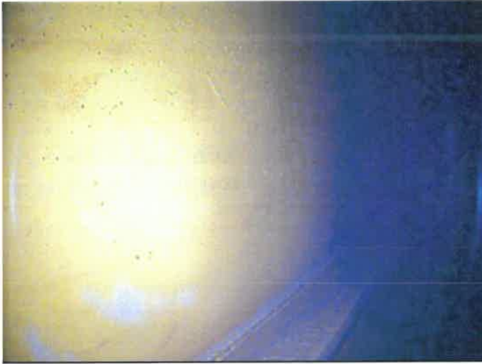
55) Coating blisters above the sidewall stiffener ring.
