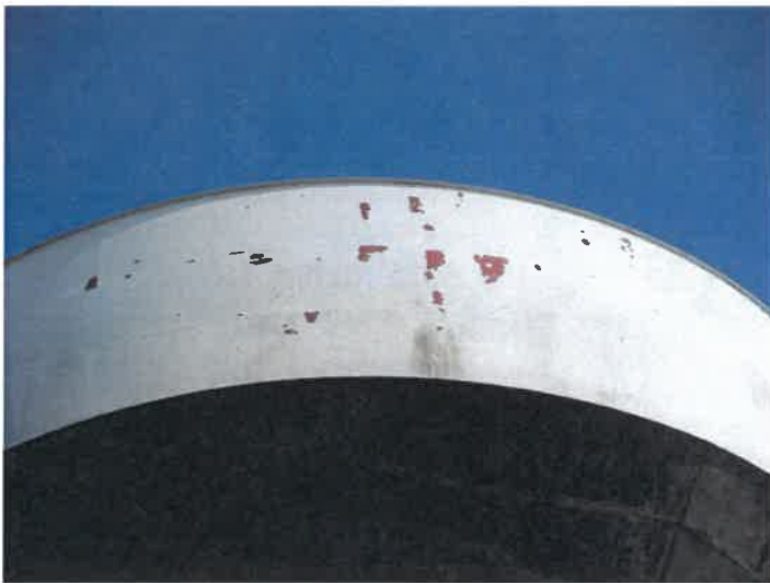
16) Coating delamination on the sidewall.
