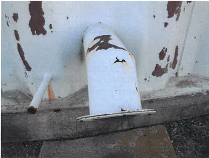
10) Coating failures on the overflow pipe.
