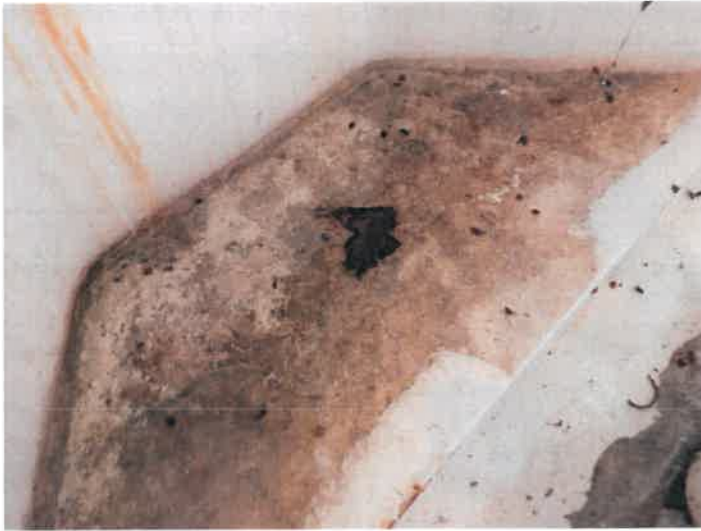
31) Spot coating failure on the baseplate in the dry interior.
