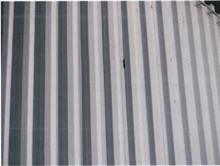
7) Spot coating failure on the column.
