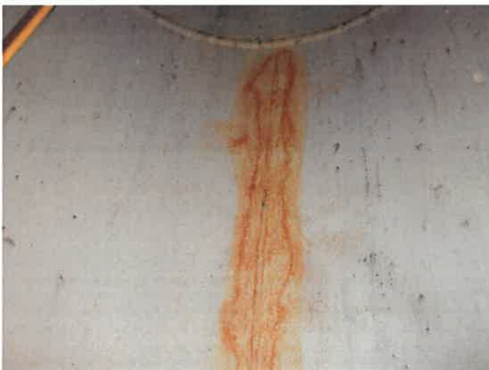
48) Spot coating failures and rust bleedthrough in the access tube.
