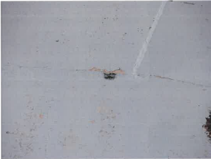
19) Spot coating failures on the roof.
