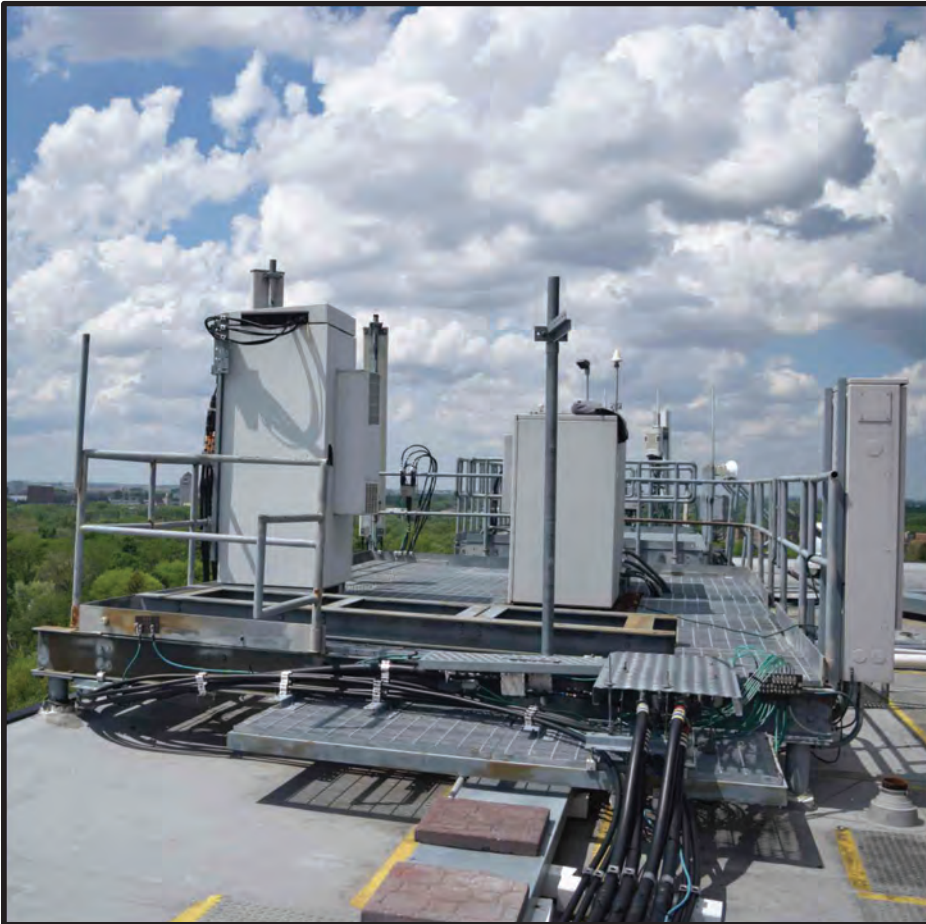
A EXISTING EQUIPMENT PLATFORM COAX ROUTING
