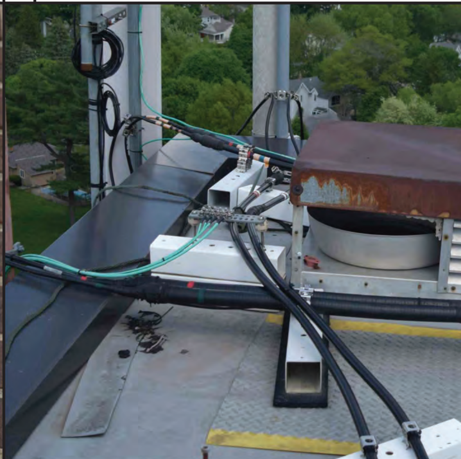
F EXISTING ALPHA SECTOR GROUND BAR
