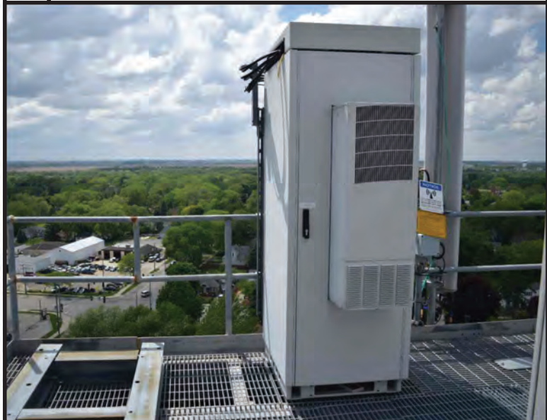
D EXISTING LTE CABINET TO BE REMOVED
