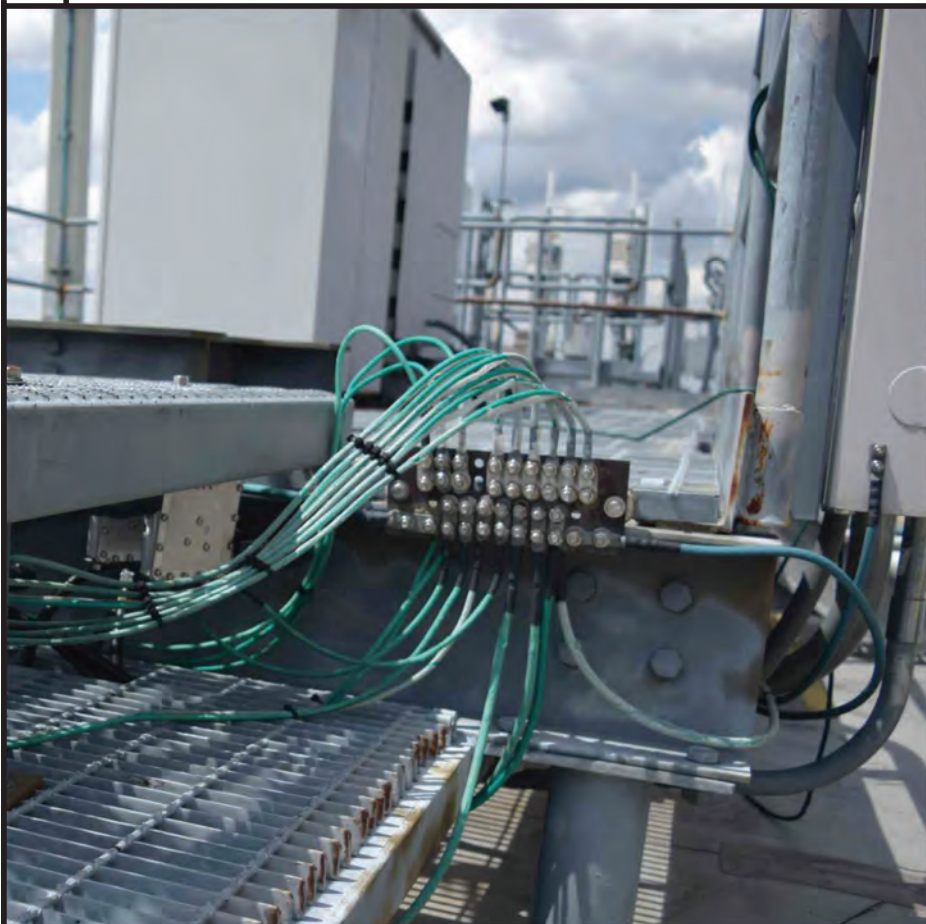
D EXISTING EQUIPMENT GROUND BAR
