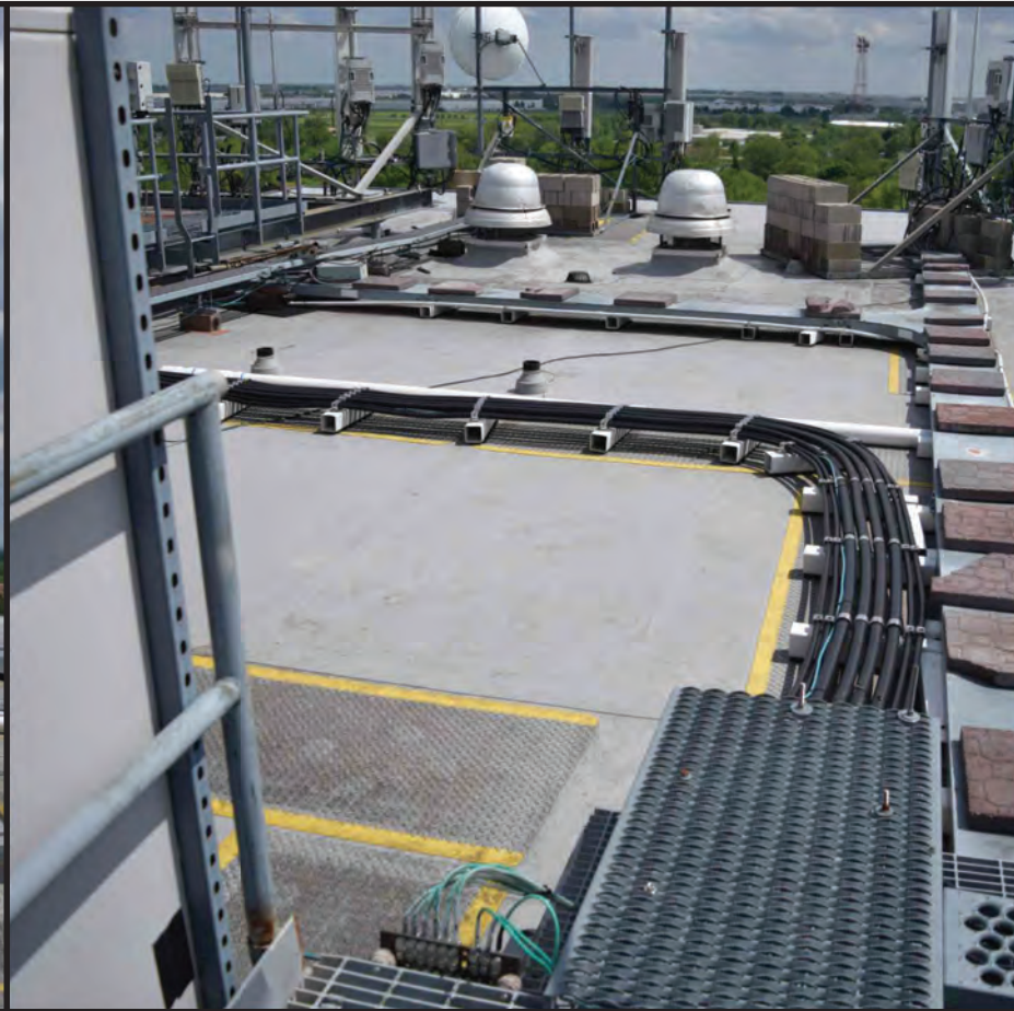
B EXISTING COAX ROUTING
