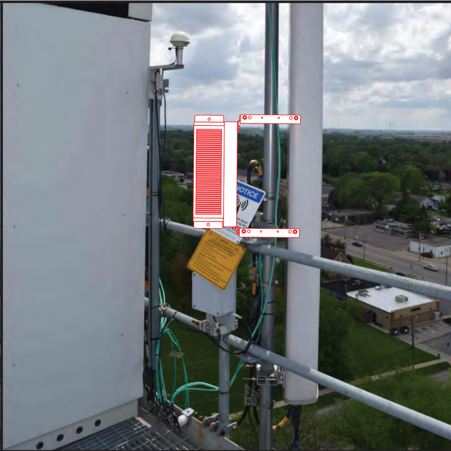
B PROPOSED RADIO EQUIPMENT LOCATION @ PLATFORM
