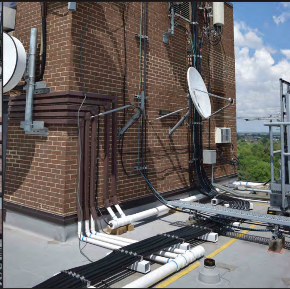
C EXISTING COAX ROUTING TO BETA & ALPHA SECTORS
